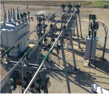
Close-up of GreenJacket installed.
