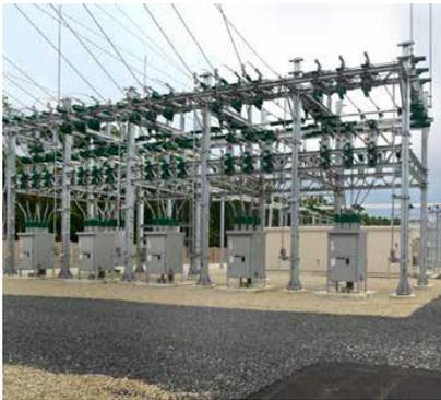
The new Franklin Township distribution substation utilized Greenjacket® precise fit cover-up as an integral part of their avian protection plan.
