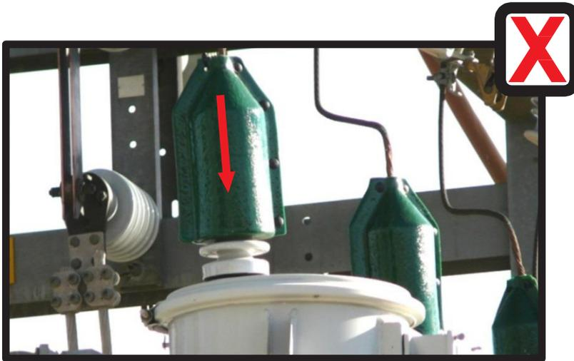
Incorrectly installed product over multiple sheds
